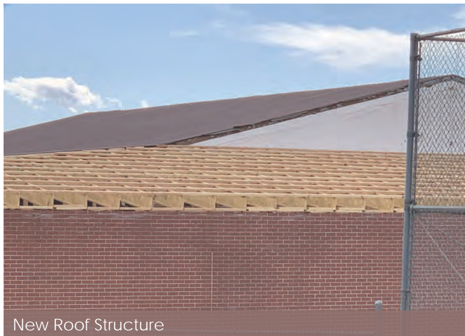
New Roof Structure
